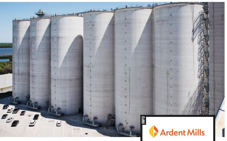
The 160-foot (around 50 meters) silos have a total storage capacity of 111,000 tonnes.
