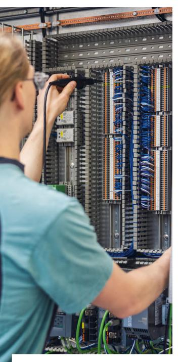
A Bühler inspector carries out a functional check on a control cabinet, in this case a five-roll refiner retrofit for chocolate.
