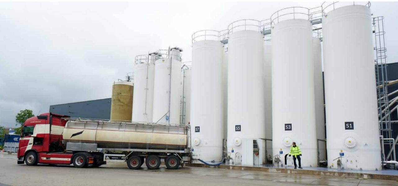
The organic residues are stored in silos before they are mixed into a proper feedstock.
