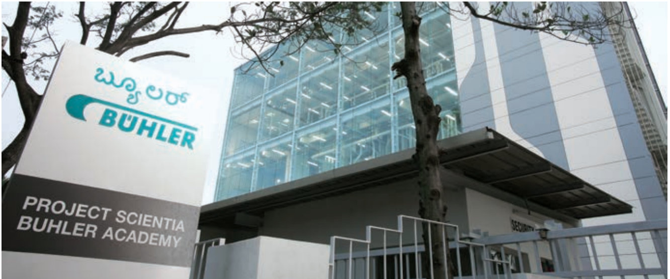
The Bühler Application Center in Bangalore for process developments, trainings and tests
